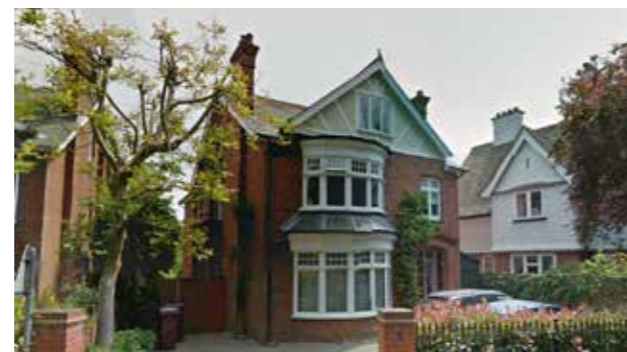
Berkshire orange brick, bay fronted house on The Mount, Caversham
